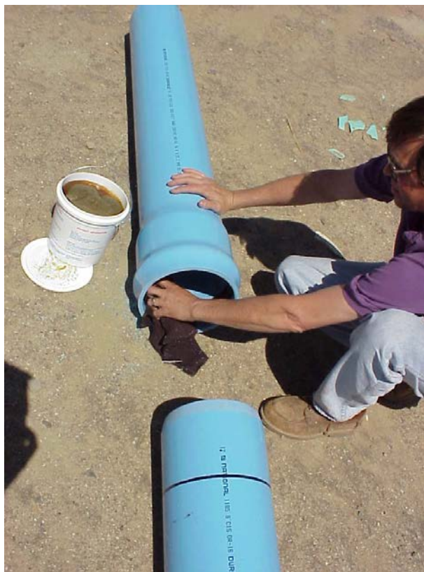
Figure 2 - Clean the bell interior and spigot
