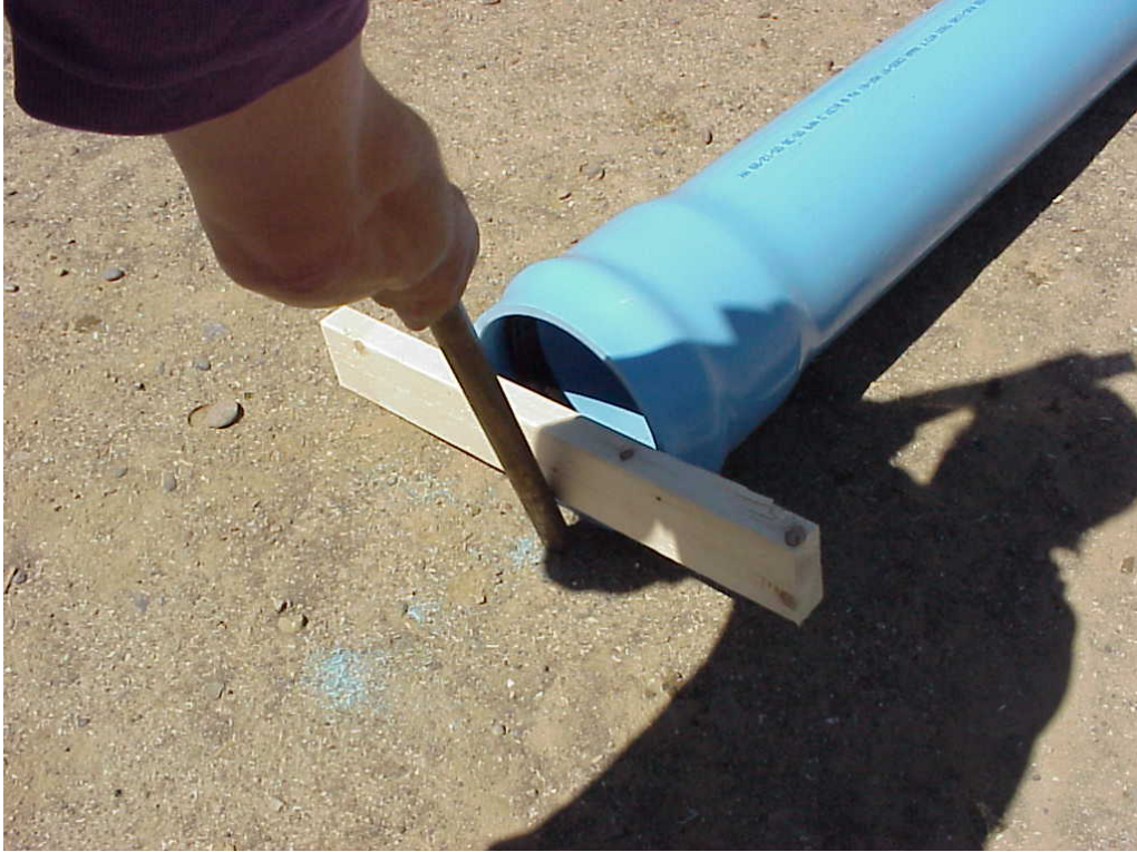
Figure 5 - Bar and block assembly
