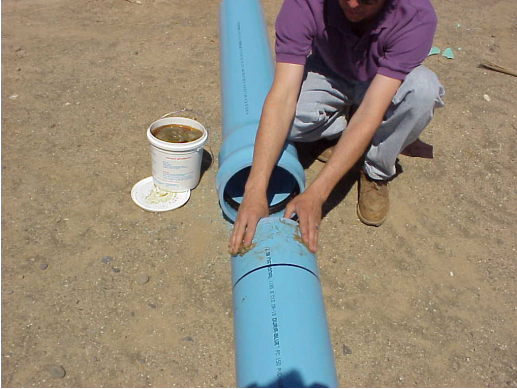
Figure 3 - Lubricate the bell, gasket, and spigot
