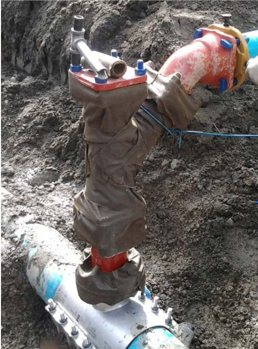
Figure 20 - ROMAC SST 8'x4' Tapping Sleeve w/restrained riser
