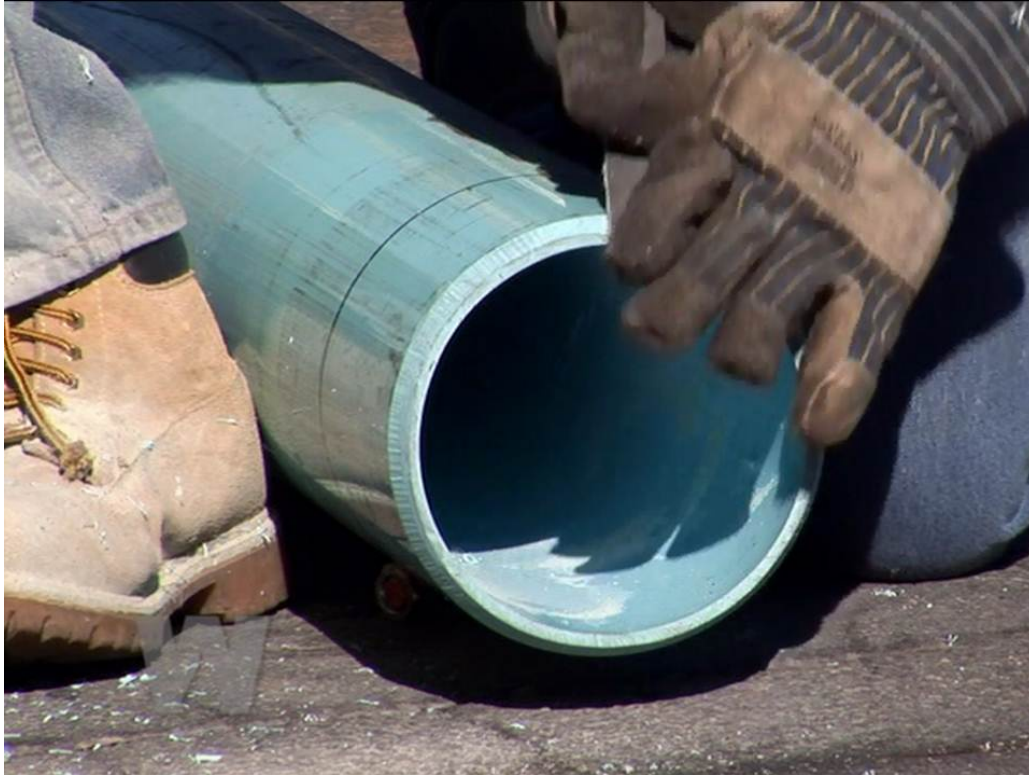
Figure 12 - Remove any burrs and smooth out rough areas
