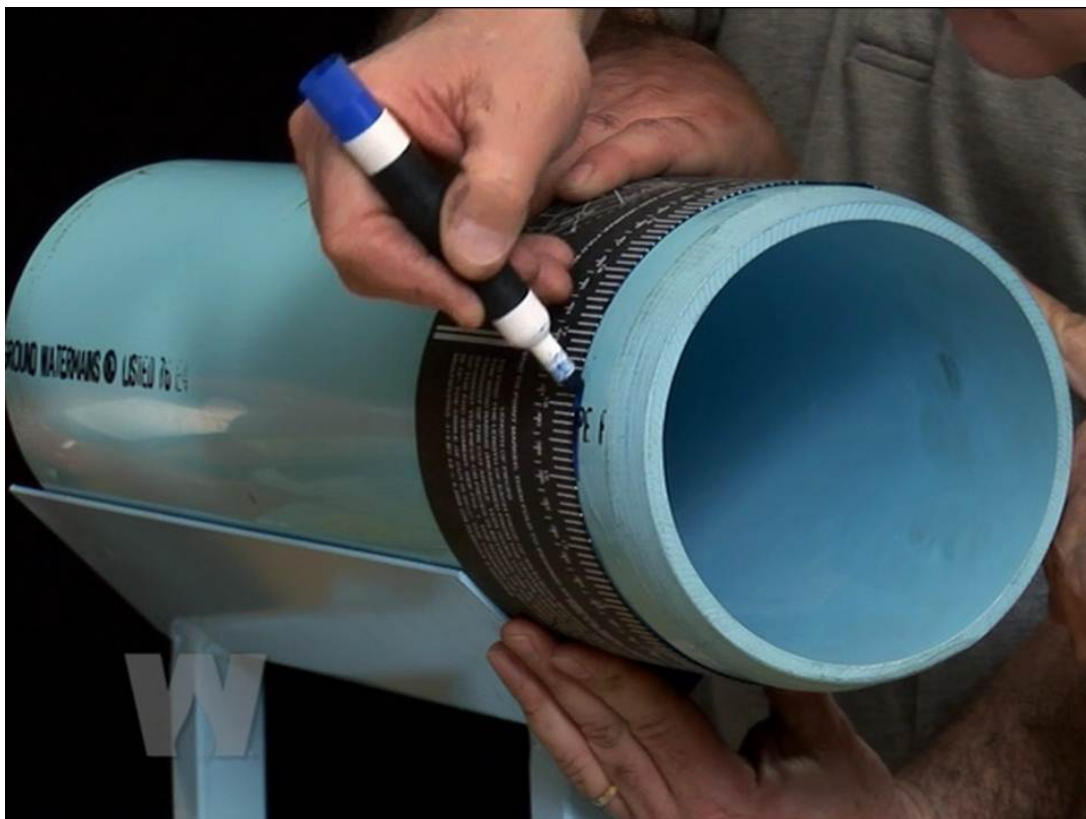
Figure 13 - Add a new insertion reference mark
