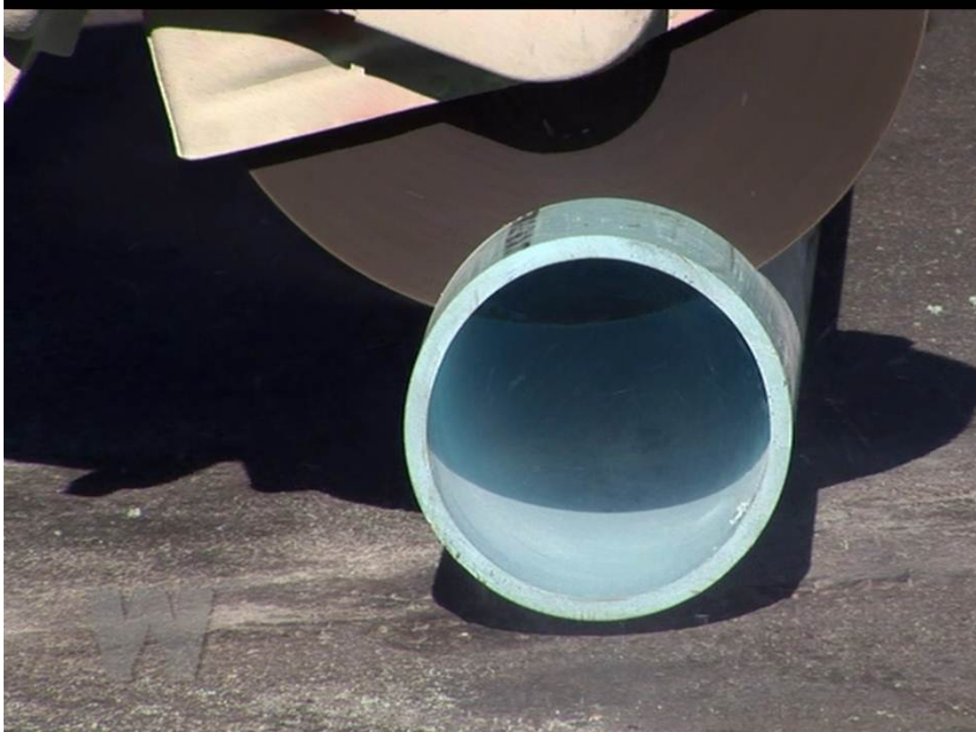
Figure 10 - Cut the pipe square
